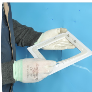
Place the seal over the flange
